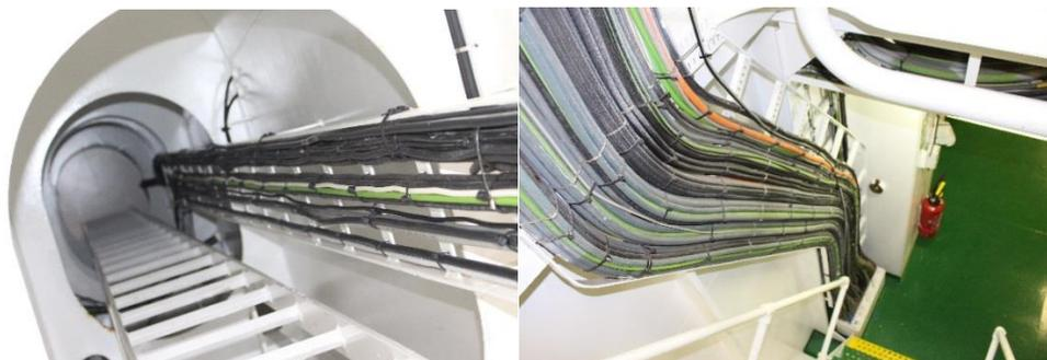
**Figure 12:** Air inlet line and GPS cable running through the cable pathway.
